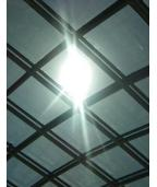
The results of the testing revealed that the transmission of UV and visible light through the as-built glass conformed to the specified levels. In addition, WJE did not detect any locations of UV or visible light concentration under the dome. Thus, WJE concluded that the glass panels performed in accordance with the approved design.
